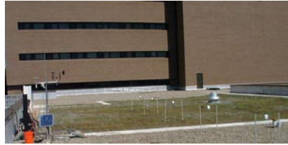
Photo courtesy of Angie Durhman. PSSB green roof on August 28, 2004 equipped with monitoring instrumentation. Cement pavers separate the gravel ballast from the vegetated section.
